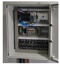
A PLC controls all of the field devices required for full weighbridge operation. This would usually consist of traffic lights, position sensors, alarms, etc.
